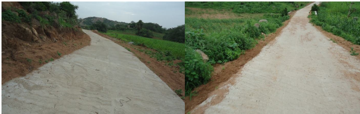
The road constructed by BDL
